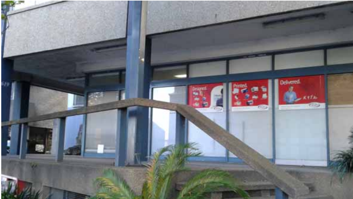
Photo 3 – View of ground floor of Building 619
