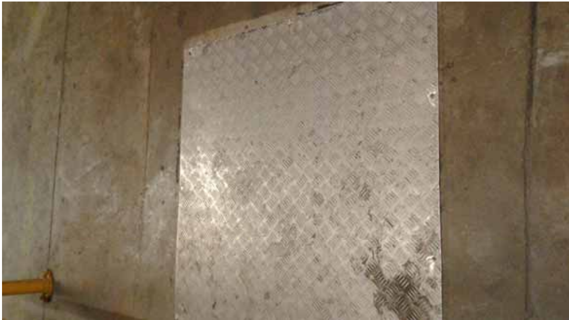
Photo 7 – View of underground rainwater system
