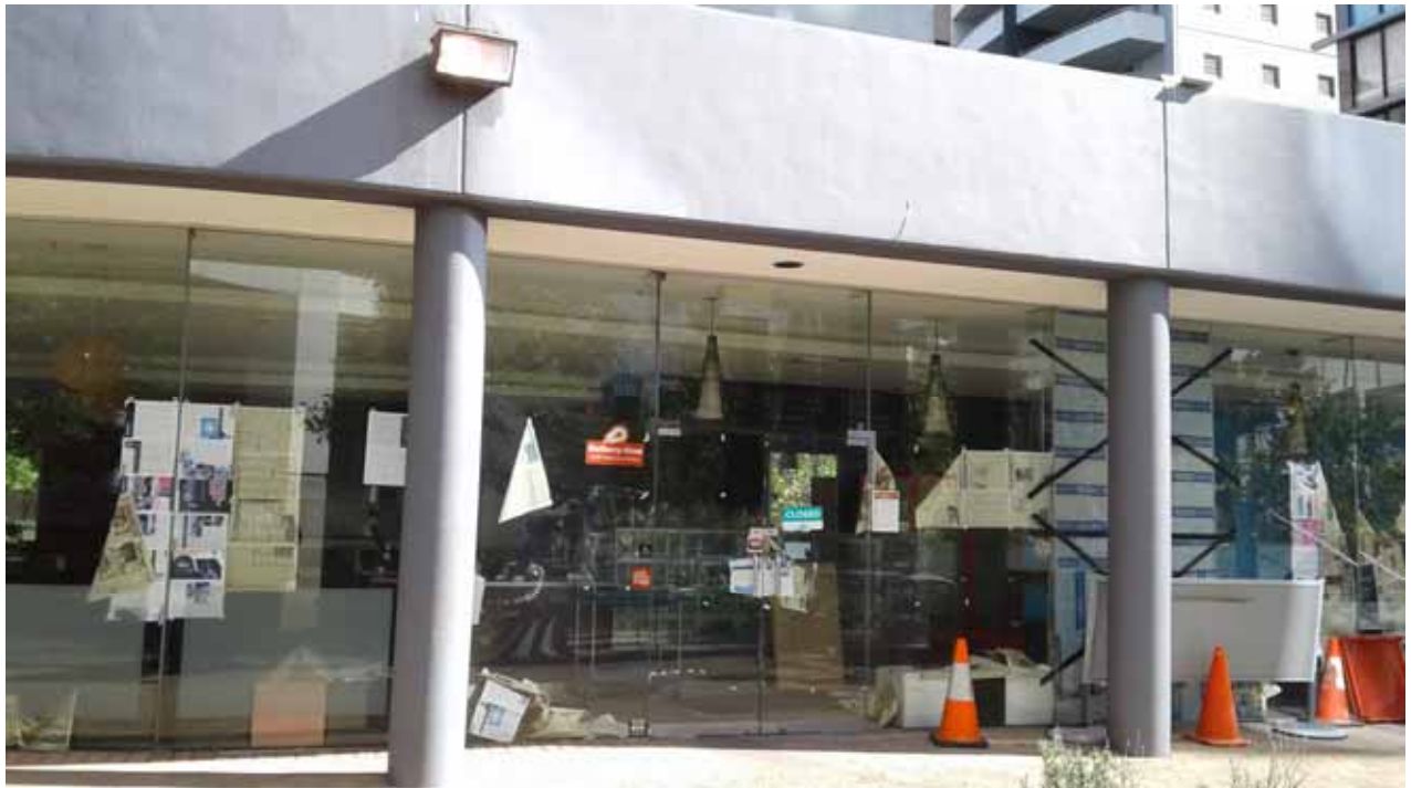
Photo 4 – View of ground floor of Building 619
