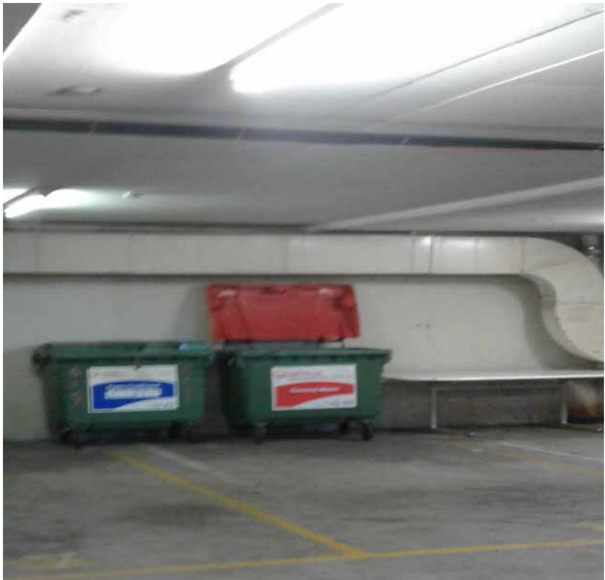
Photo 18 – View of rubbish bins and rubbish chute
