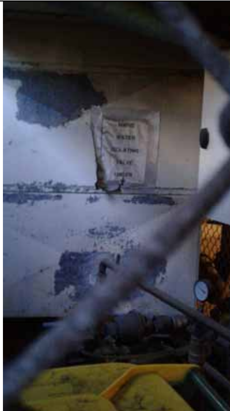
Photo 15 – View of storage 2
